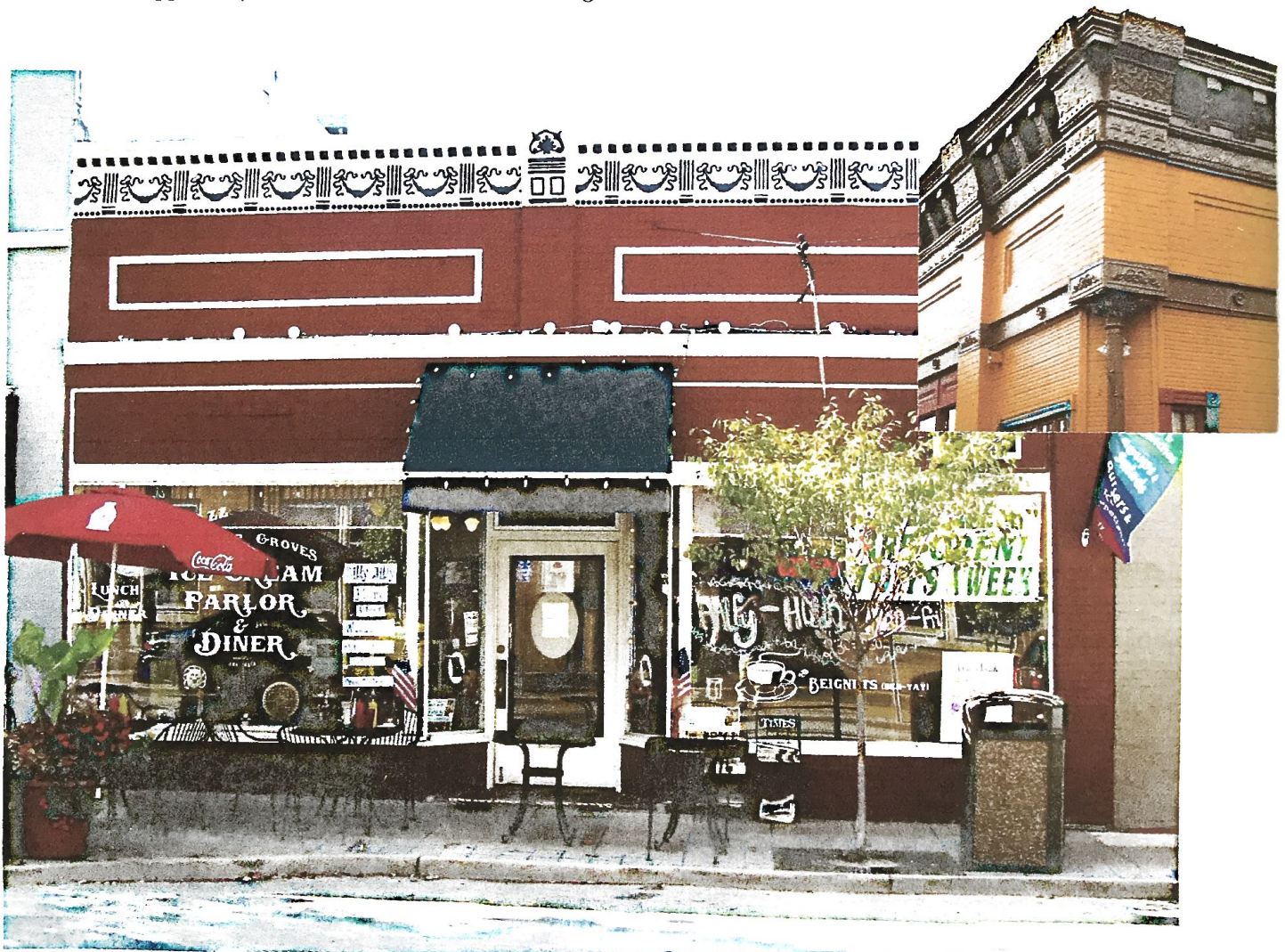
Pressed metal cornices manufactured from two different Mesker factories are side by side in Webster Groves, Missouri. Photographs by Jim Winnerman, 2012.
